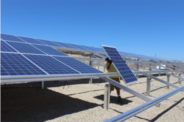
Panels can be inserted from underneath the array
